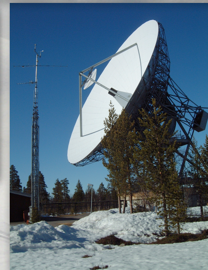
Tristatic UHF, 930MHz
